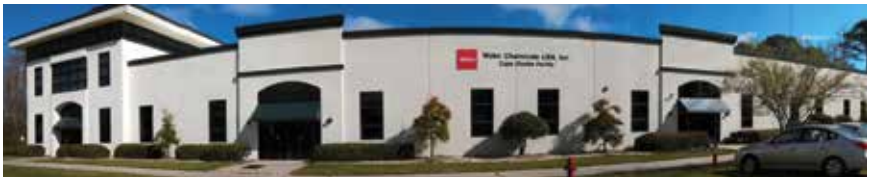
FUJIFILM Wako Chemicals U.S.A. Corp. - Cape Charles Bleeding Facility: Cape Charles, Virginia 23310
