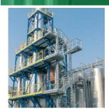
Solvent recovery from waste streams through the combination of mass and heat transfer in specialized columns.
