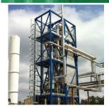
Recovery of VOCs through cryogenic condensation. This customizable and flexible process is suitable for most VOCs.
