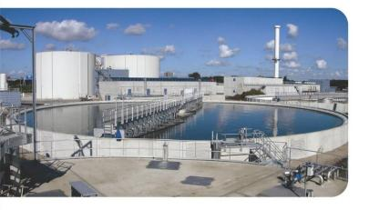
Apurva Water design, manufacture, supply and provide the services for the Sewage Water Treatment Plant and Effluent Water Treatment Plant. The system is designed to work on high MLSS and low HRT by using the state of art technology MBR that is Membrane Bio Reactor Which is highly sophisticated and less complicated.
