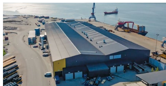
Freyr Battery is perfecting its manufacturing process at this site in Mo i Rana, Norway.
