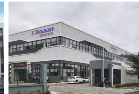
Canaan Kaixinlong Factory
