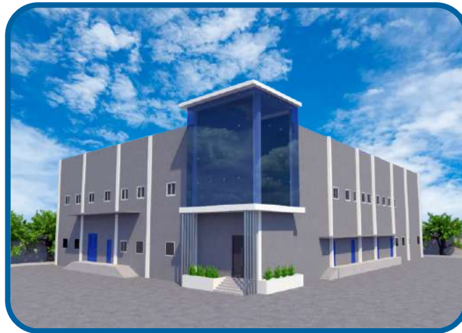
Unit-2 Oncology Injections
