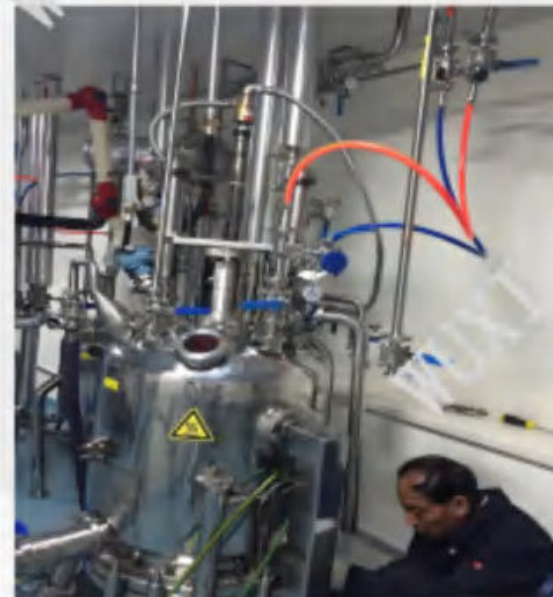
On site commissioning DN500 ANFD
