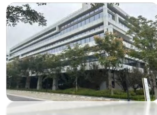
MFG2 Nanjing Manufacturing Site (9,000 m 2 )
