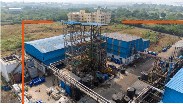
Effluent Treatment Plant
