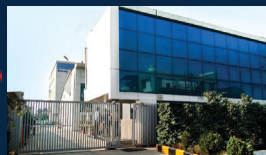
API Facility I ANKLESHWAR, GUJARAT
