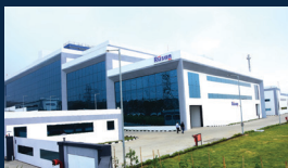
API Facility II PITHAMPUR, MADHYA PRADESH
