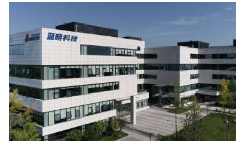
Sunresin Park, Headquarter
