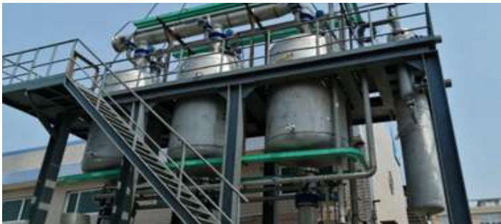
Toluene treatment project, Zhejiang (10000m 3 /h)
